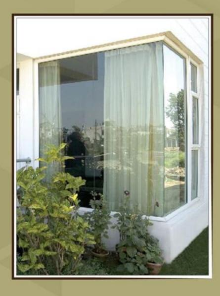
Glass-to-Glass Window features a fixed window unit, where the glass panes meet at an angle of 90° and are neatly joined together without using any mullions.
